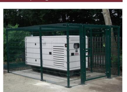
shenton**group** have developed a practical and cost effective security package to prevent increasing vandalism and malicious damage. This package includes a strong steel mesh security cage. All steel work is galvanised and then polyester powder coated for longevity of life. The mesh is constructed from mild steel 6.0mm vertical wires sandwiched between 2no 8.0mm horizontal wires, with 200x50mm
