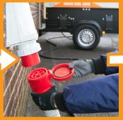
A weatherproof plug and socket provide fast and safe connection to your premises.
