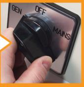
A manual changeover switch allows selection between mains power and generator.
